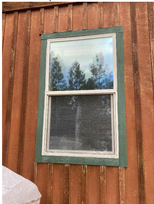
Torn Window Screen (typical of 2 first floor windows this elevation)
