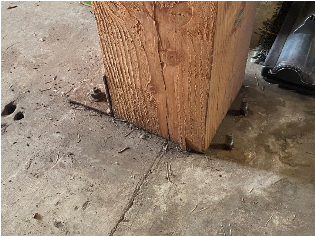
Inadequate Post Connection to Slab
