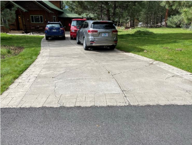
Cracked Driveway Surface
