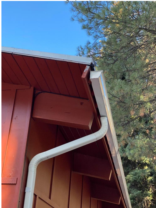
Roofing Close to Failure at Gutters
