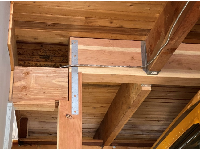
Inadequate Post to Beam Connection
