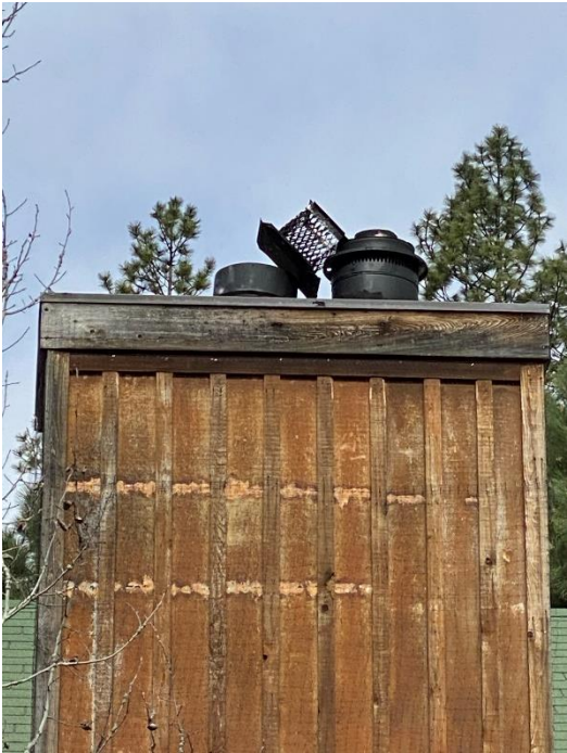
Chimney Spark Arrestor to be Secured
