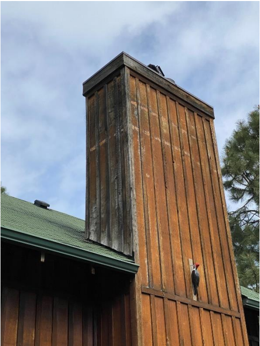
Siding Damage on Chimney
