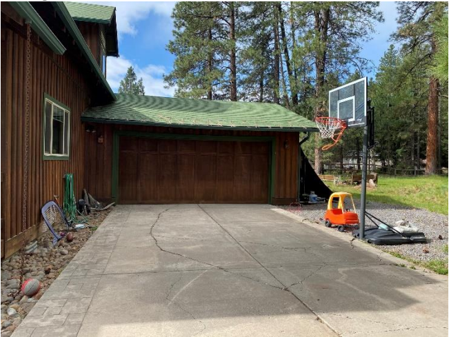
Cracked Driveway Surface & Sagging Roof over Garage Door
