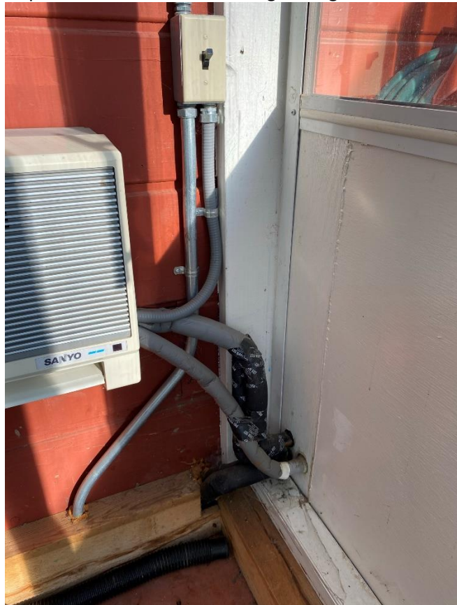
Unprotected Access to Plumbing-Wiring
