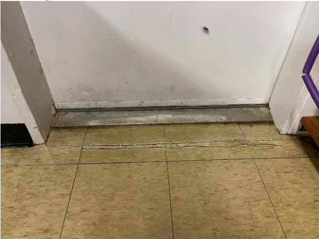
Cracking Floor Tiles
