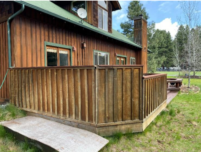
Deck Wall Enclosure Failure at Corner and Needs Re-Finish
