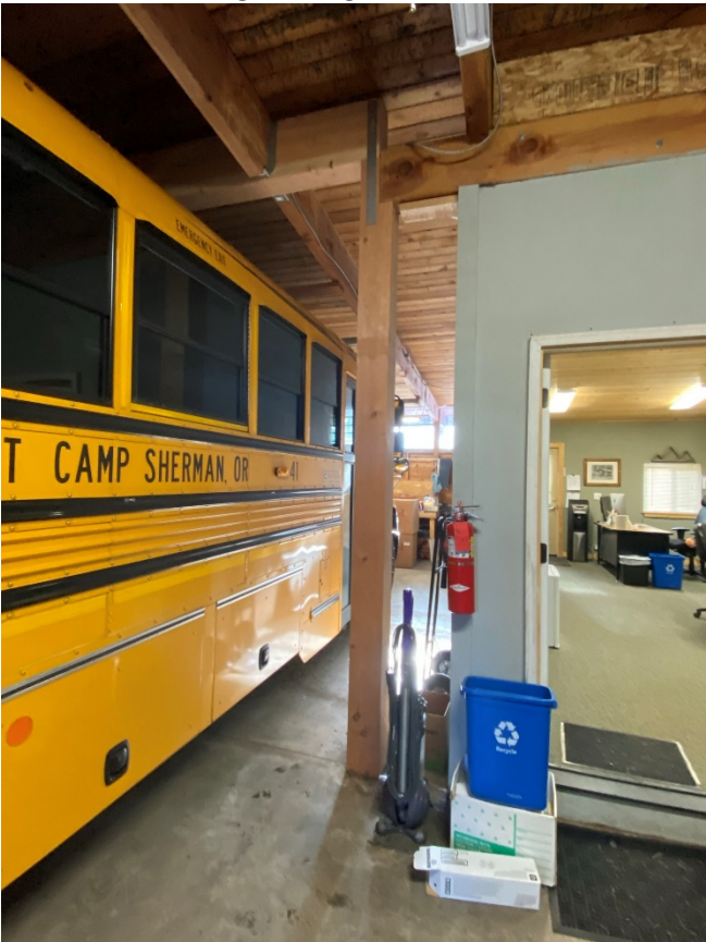
Inadequate Post to Beam Connection
