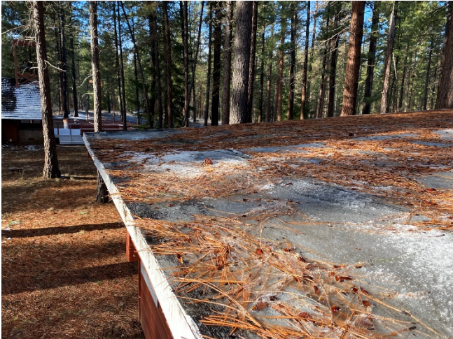
Ice & Debris in Internal Gutter
