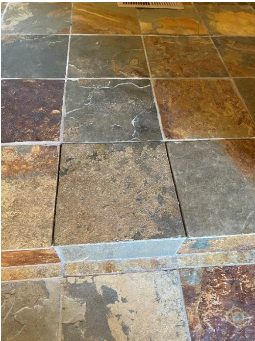
Entry Slate Tile Floor – Missing Mortar
