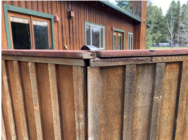
Closeup of Deck Wall Corner Failure
