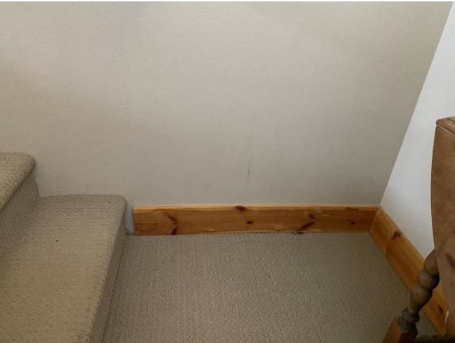
Stairway Baseboard Missing at Stairs
