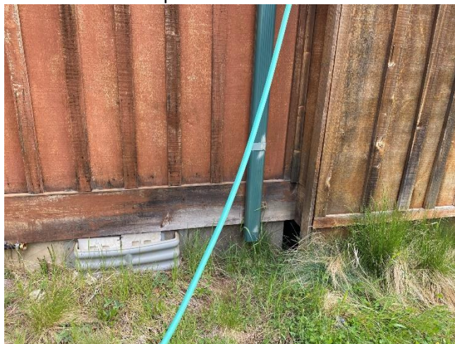
Siding Needs Re-finishing / Better Drainage to be Provided at Downspout
