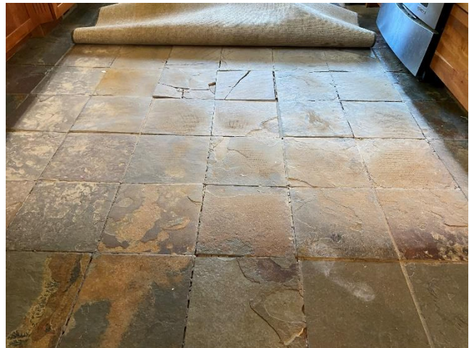
Kitchen Slate Tile Floor to be Replaced
