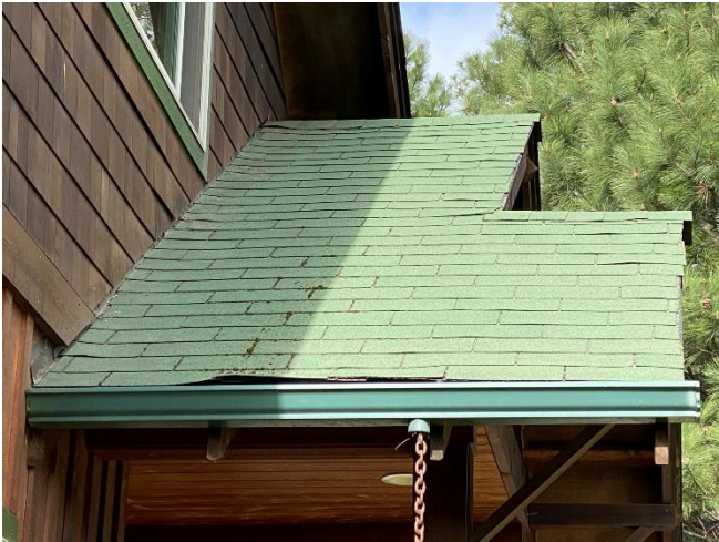
Damaged Roofing on Entry Canopy
