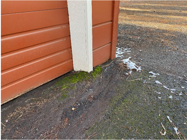
Sididng and Posts within Dirt + Drainage Issue
