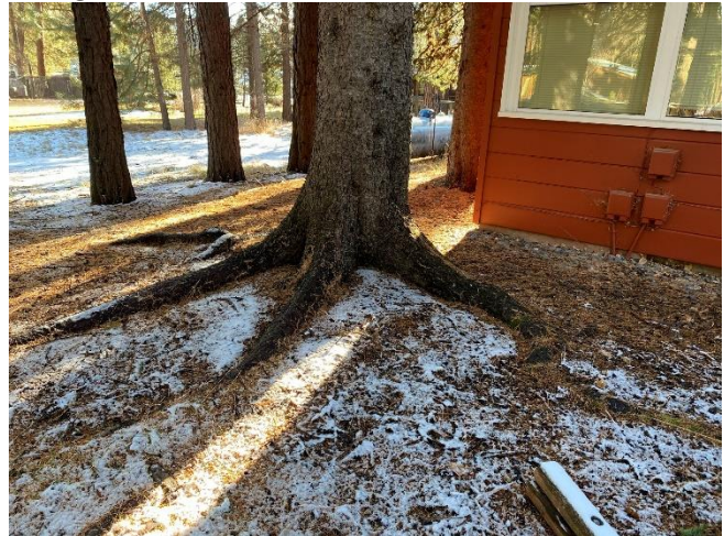
Overgrown Tree Roots close to Structure
