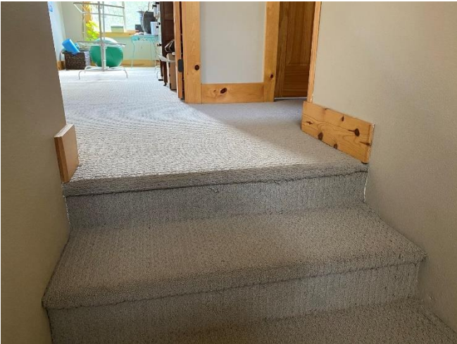
Stairway Baseboard Missing at Stairs
