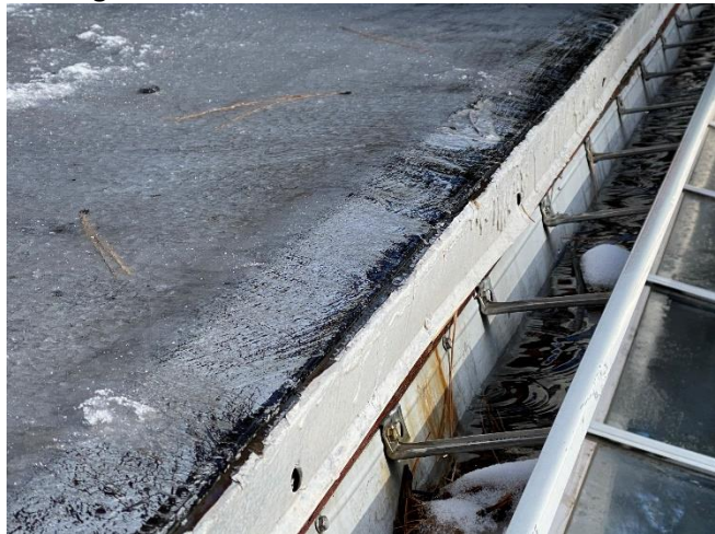
Roofing Close to Failure at Gutters
