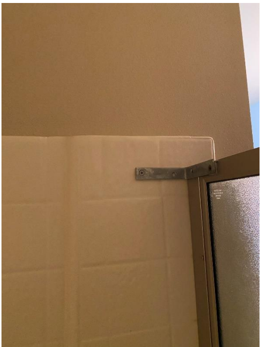
Master Bathroom Shower Enclosure Reinforcement
