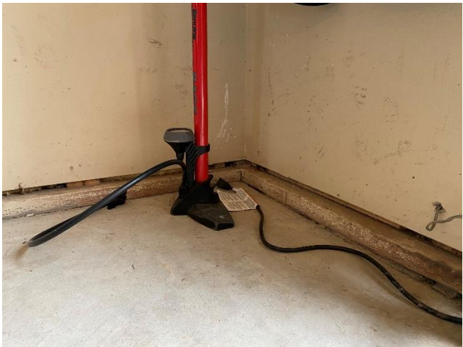
Garage Not Constructed with Concrete Curb
