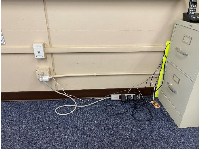
Inadequate Power Supply
