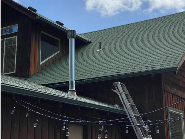
West Roof Damage along Roof Edge & Gutter Pulling off Fascia
