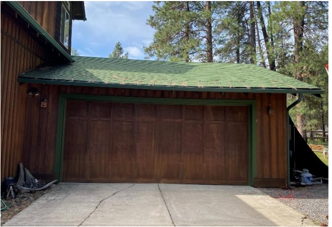
Sagging Roof over Garage Door
