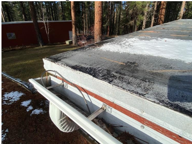
Membrane Roofing Close to Failure
