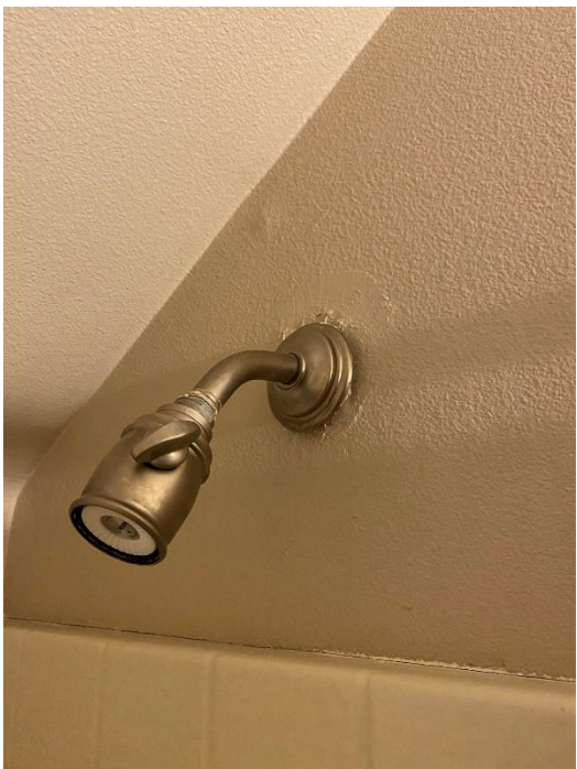
Upstairs Bathroom Faucet Not Secure to Wall
