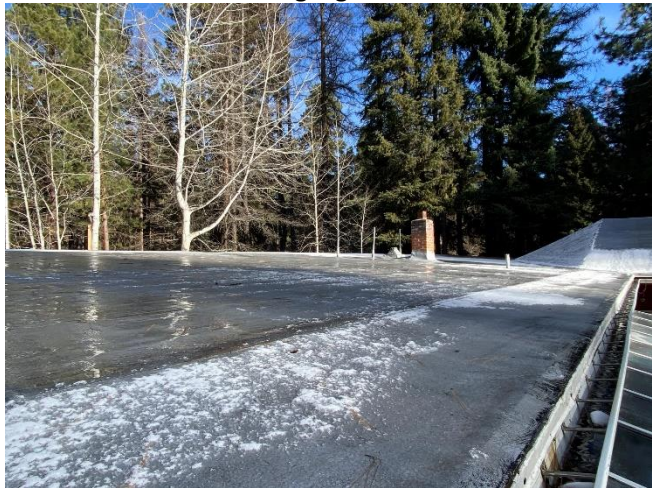
Membrane Roof Showing Significant Wear
