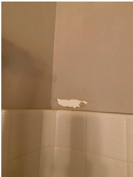
Master Bathroom Shower Drywall Damage
