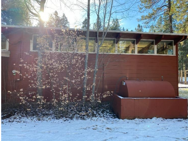
Single Pane Windows, Propane Tank Close to Building
