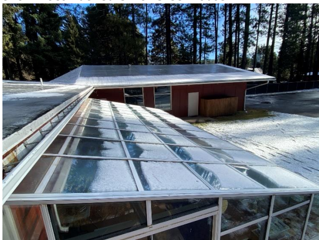
Snow Doesn't Shed Off of Greenhouse
