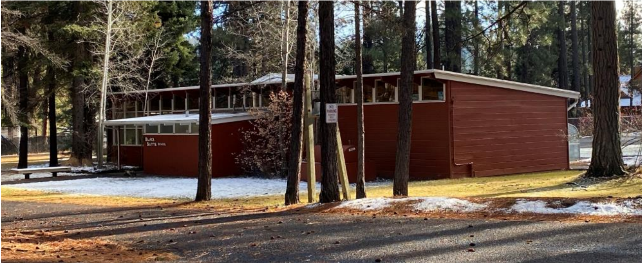
North-West (front-side) Elevation of School
