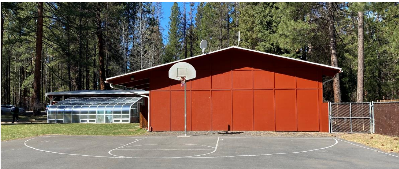
South (rear) Elevation of Greenhouse Addition (on left) and Multipurpose Room Addition (on right)
