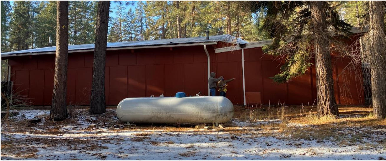
East (side) Elevation of School (on right) and Multipurpose Room Addition (on left)
